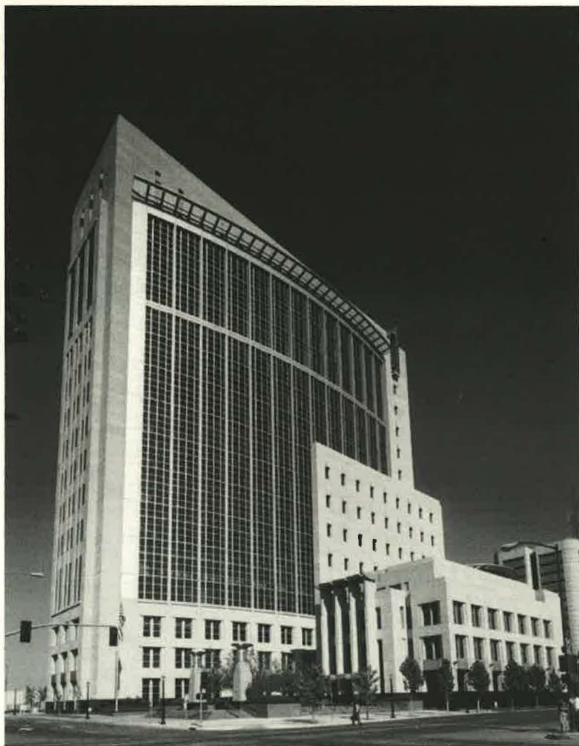
Matsui Courthouse, Sacramento, exterior
